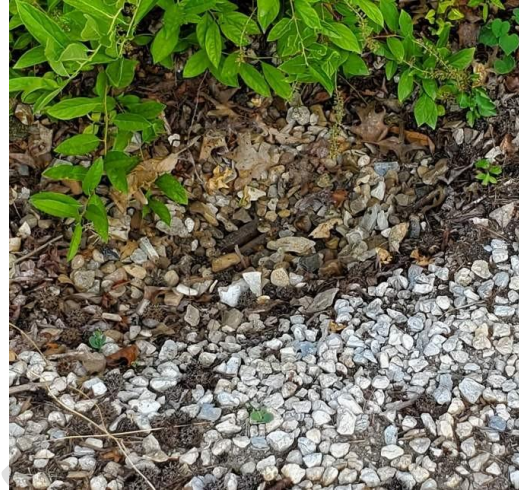
East flower bed inlet overgrown, covered with rock.
