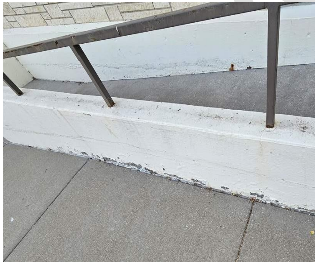
Entry Ramp Railing
