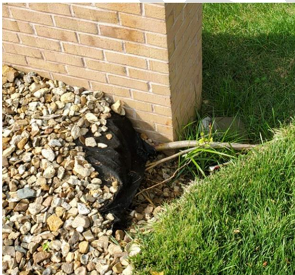
Northwest corner of building at screen wall.
