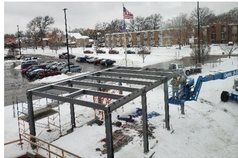
Even with the poor weather, crews have made progress on the pavilion and the trellis. Masons have started laying cinderblocks for the walls of the pavilion and the top support structure of the trellis has been installed.
